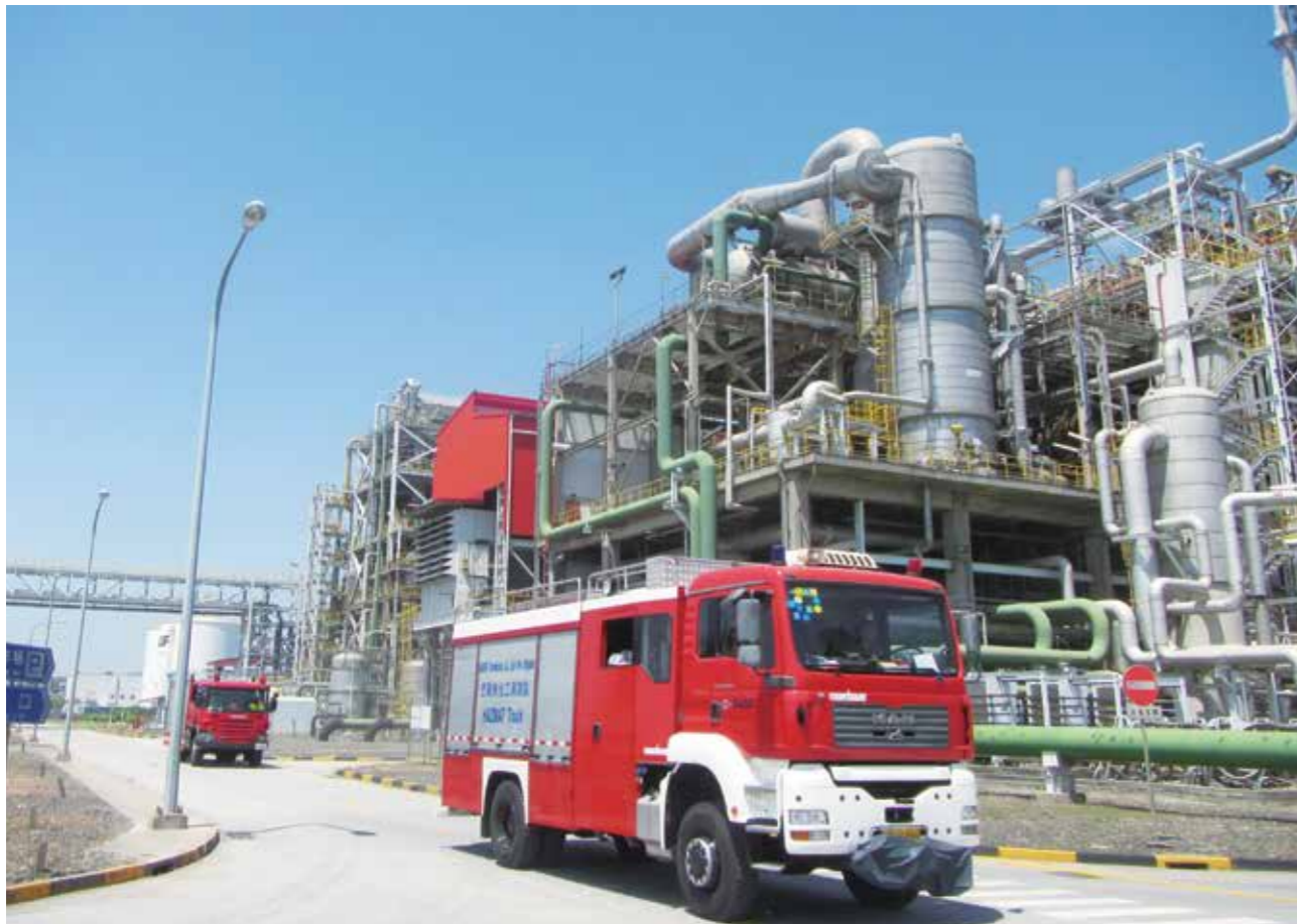
The BASF fire brigade at Caojing site in Shanghai conducts regular emergency response training.
